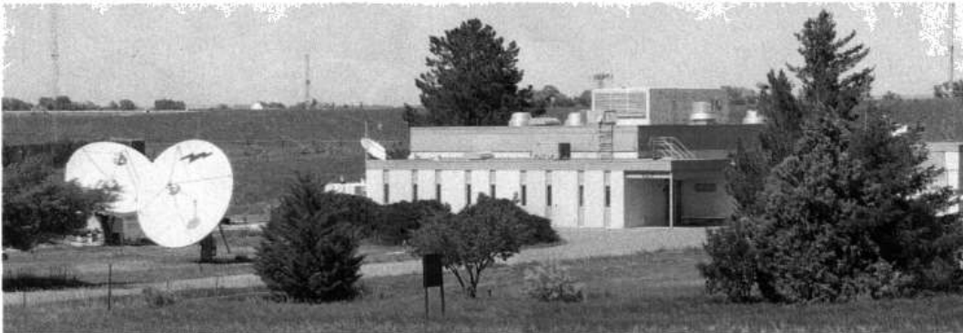
Timing, signal-generation, and transmitting equipment can be found in the radio station's main building.
