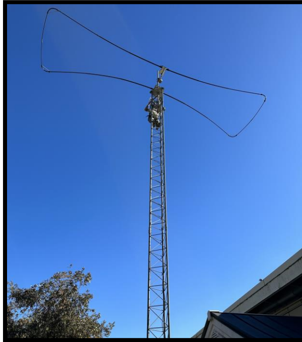
Eric KE6MLF doing tower work at KJ6LV
