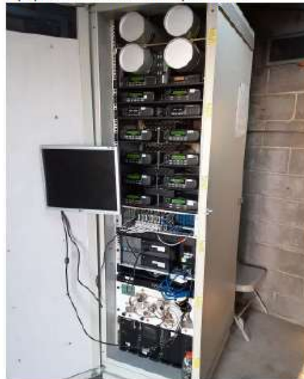
Equipment installed and operational
