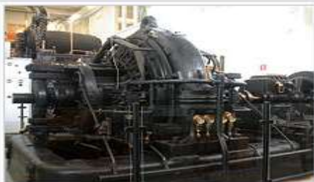
200 kW Alexanderson alternator preserved at the Grimeton radiotelegraphy station, Sweden, the only remaining example of an Alexanderson transmitter.
