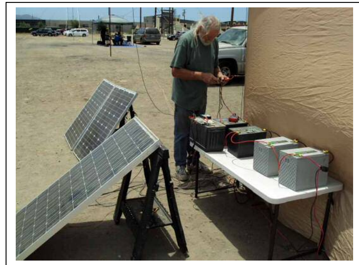
John Gartman AG6GL at the 20M SSB Solar/Battery array – photo de K6NE
