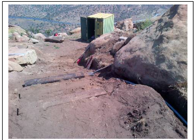
Conduit and access stairs
